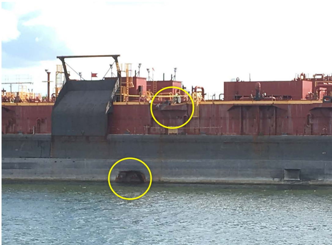
Damage to OSG 243 , port side. Yellow circles identify, at top, cantilever deck damaged by Yochow 's bow rake and, at bottom, side shell at waterline in no. 5P ballast tank penetrated by bulk carrier's bulbous bow.
